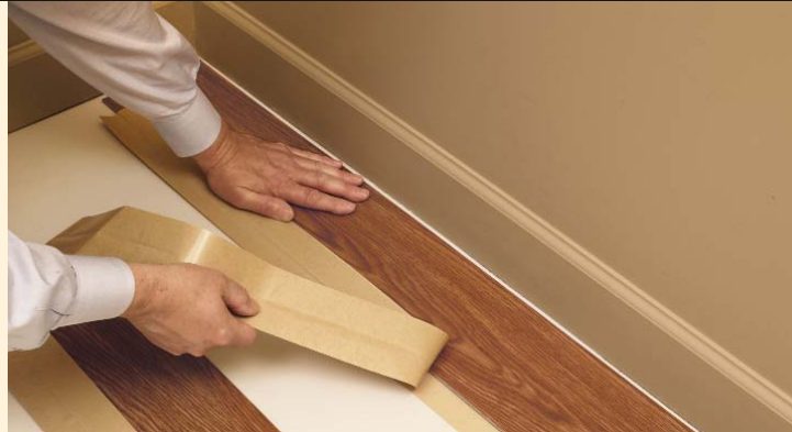
Install first row parallel to the longest wall and remove the release paper.
