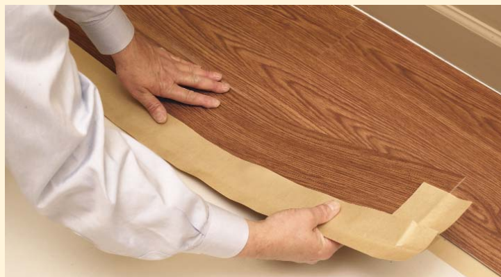
Continue installing planks.
