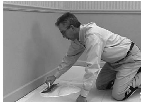
Fig. 6. Apply adhesive and install product.
