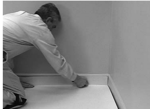
Fig. 4. Cut leaving 1/8" to 1/4" space at perimeter.
