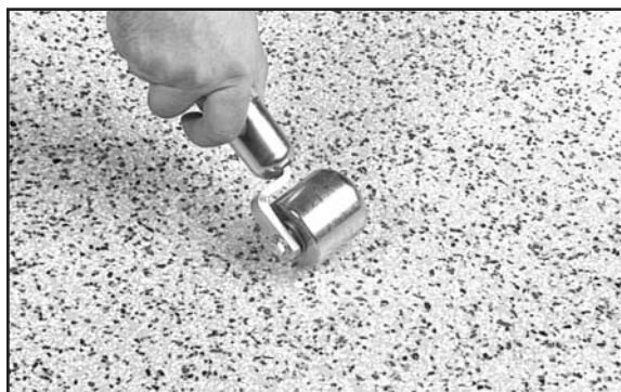
Fig. 33. Roll top sheet into place with a steel hand roller.
