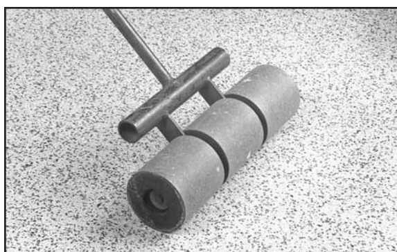
Fig. 34. Roll seam with a 100-pound (45 kilogram) floor covering roller.
