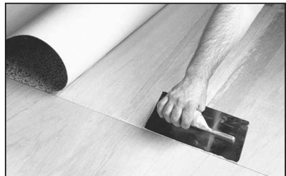
Fig. 28. Carefully spread adhesive up to the guide line.
