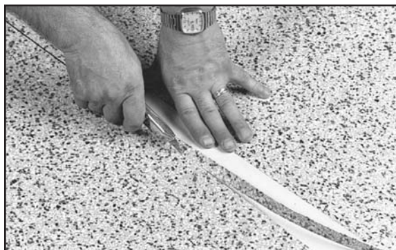
Fig. 32. Cut the seam on a 90° angle following the score marks.
