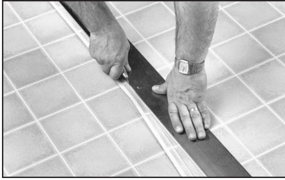
Fig. 20. Hold utility knife on 90° angle and apply sufficient pressure to cut through both layers of flooring material.
