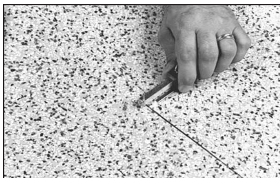
Fig. 31. Lightly score the surface of the top sheet.
