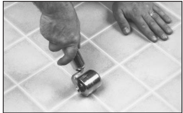
Fig. 23. Bring wearlayers level with steel hand roller.
