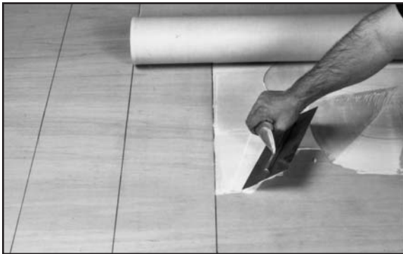
Fig. 17. Spread adhesive to first line.
