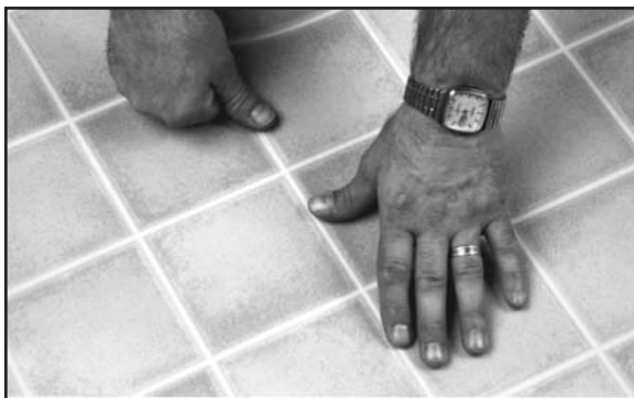
Fig. 22. Tuck sheet into place by bending slightly.
