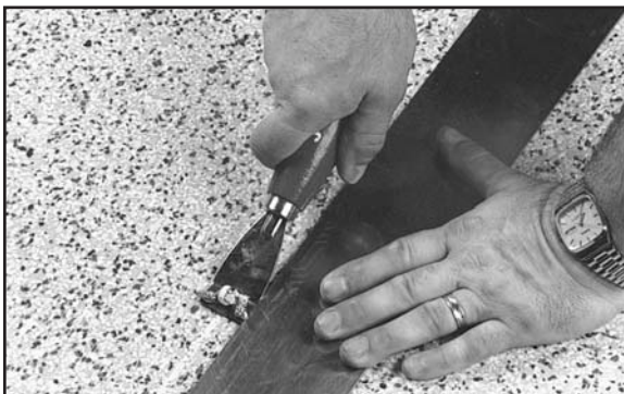
Fig. 44. Use a straightedge as a guide when using a hand grooving tool.
