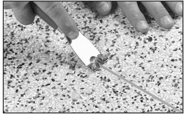
Fig. 50. Cut a tapered groove at the joint of the rods.
