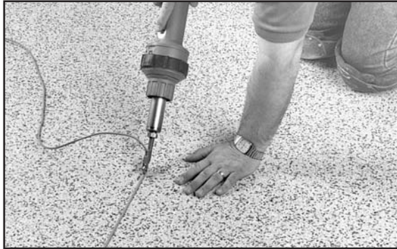
Fig. 49. Apply firm pressure while moving at constant speed.
