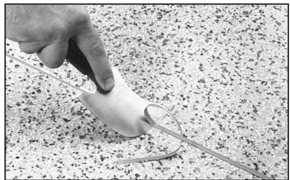
Fig. 52. Use a sharp spatula knife to produce a smooth finish.
