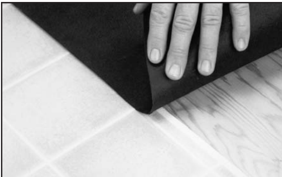
Fig. 86. Lay edge of felt even with one side of grout line.
