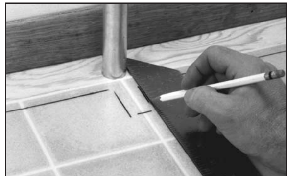
Fig. 68. Extend set marks on each side of pipe to scribe mark in front of pipe.
