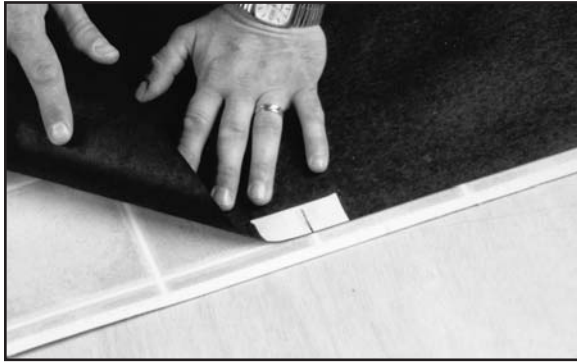
Fig. 90. Match design with mortar joints.
