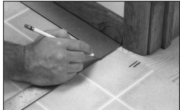
Fig. 66. Make set marks at each offset on trim pieces.
