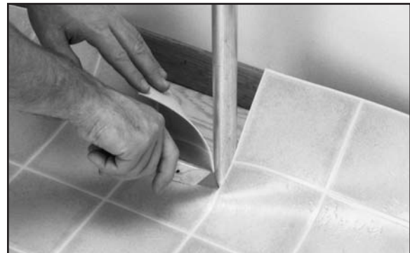
Fig. 56. Make cut to floor/object juncture.
