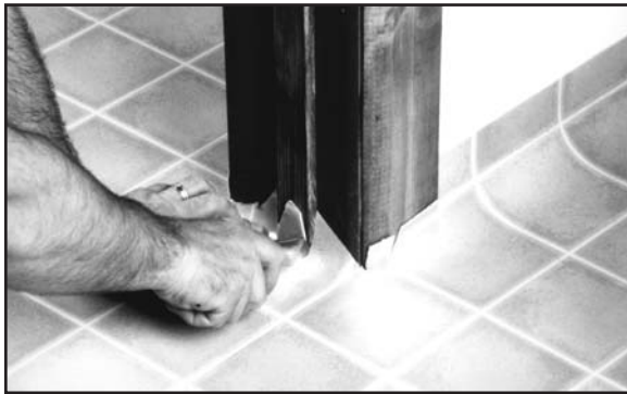
Fig. 59. Make relief cuts from top of flooring to trim/floor juncture.
