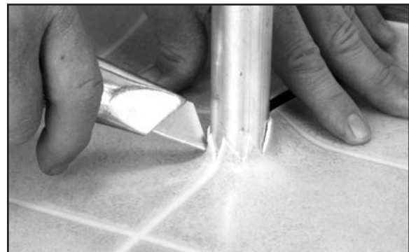
Fig. 57. Make relief cuts around pipe or object.
