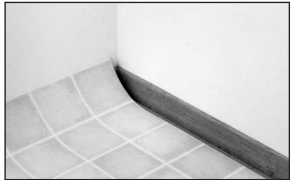
Fig. 61. Position the flooring so both ends lap up the walls.
