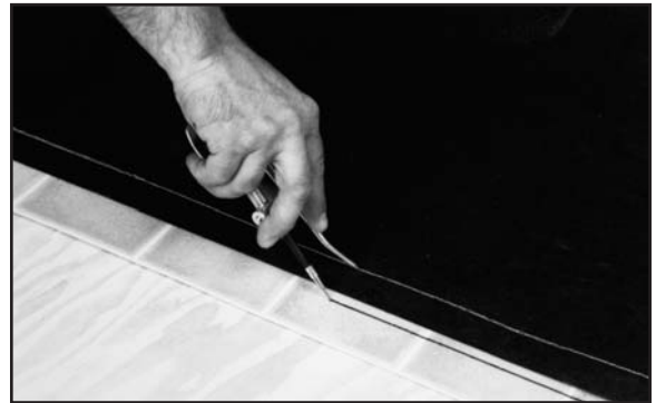
Fig. 82. Apply enough pressure against marking pin to score flooring surface.
