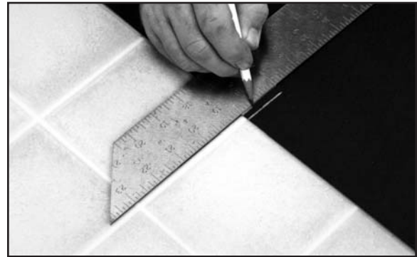
Fig. 88. Design with mortar joints: score felt where joints run perpendicular to seam.
