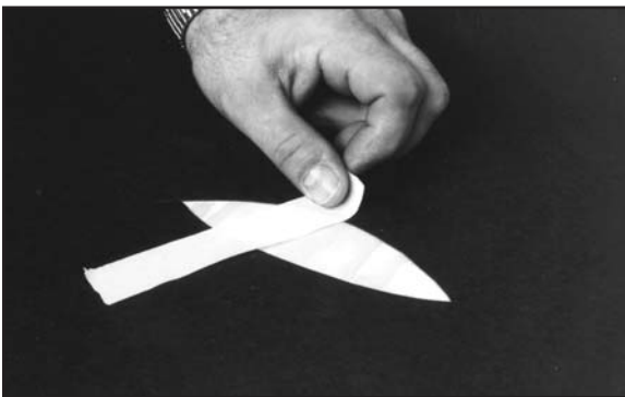
Fig. 74. Cut out oblong windows to tape felt in place on subfloor.
