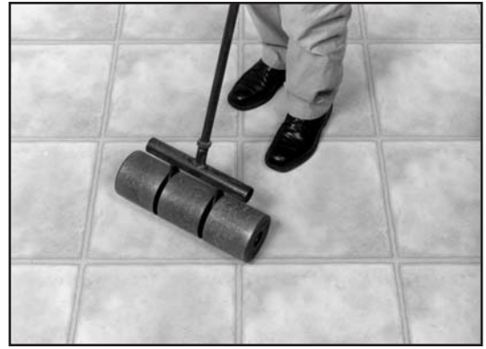
Fig. 156. Roll with a 100-pound (45 kilogram) floor covering roller
