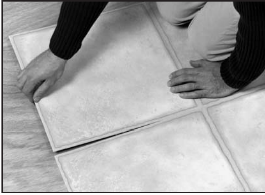
Fig. 155. Position tile at a low angle.
