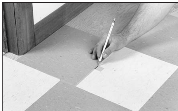
Fig. 169. Make mark on last whole tile following edge of tile being fitted.
