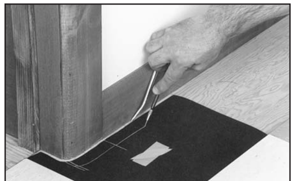
Fig. 172. Scribe wall outline onto pattern material with dividers.
