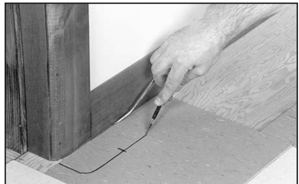
Fig. 171. Scribe wall outline onto tile; cut off excess.
