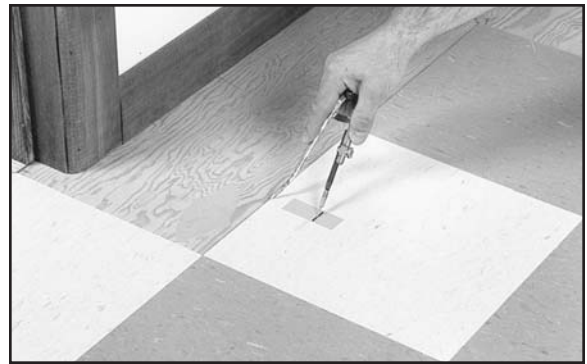
Fig. 170. Set dividers for distance between mark and tile edge.
