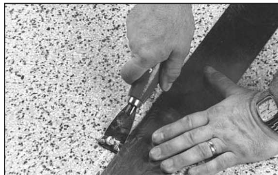
Fig. 10. Use a straightedge as a guide when using a hand grooving tool.
