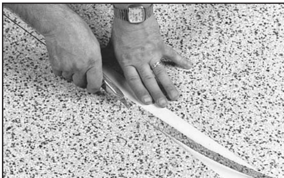
Fig. 5. Cut seam at a 90° angle following the score mark.
