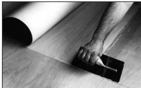
Fig. 2. Carefully spread adhesive up to the guide line.
