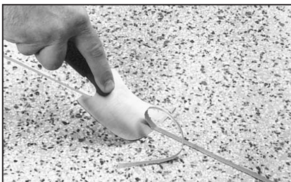
Fig. 18. Use a sharp spatula knife to produce a smooth finish.
