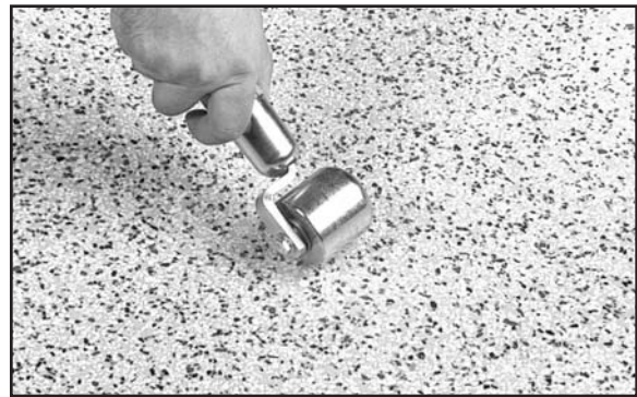
Fig. 6. Roll seam edge level.
