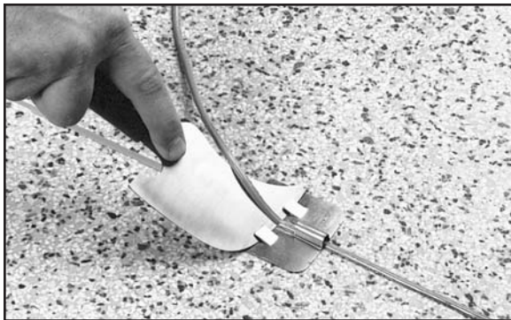
Fig. 17. Trim the welding rod using a spatula guide.
