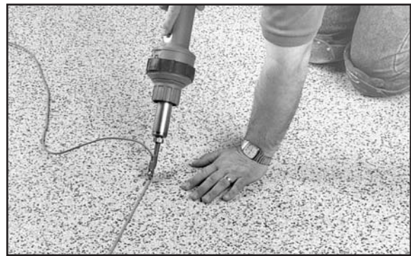
Fig. 15. Apply firm pressure while moving at a constant speed.
