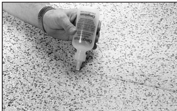
Fig. 8. Do not insert the applicator tip into the seam cut.
