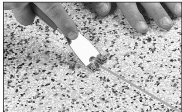
Fig. 16. Cut a tapered groove at the joint.
