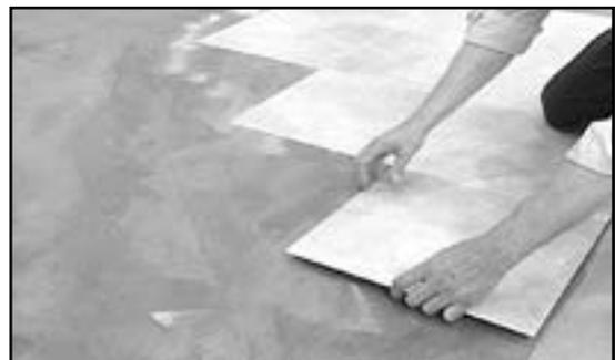
Fig. 15 - Install ungrouted floors following a stair-step pattern.
