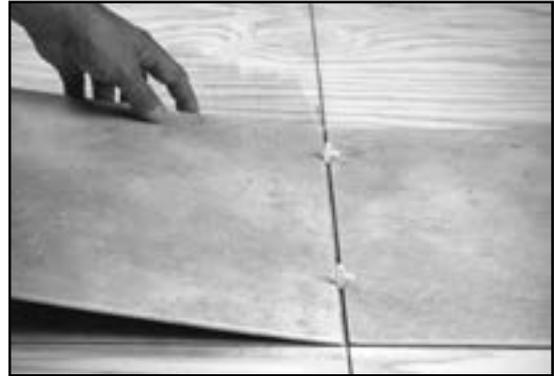
Fig. 13 - Position spacers before setting the tile.
