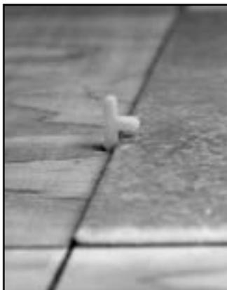
Fig. 12 - Use spacers with one leg removed.
