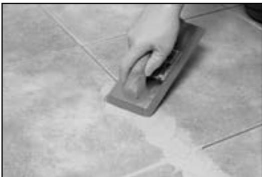
Fig. 21 - Pack the grout into the joints.
