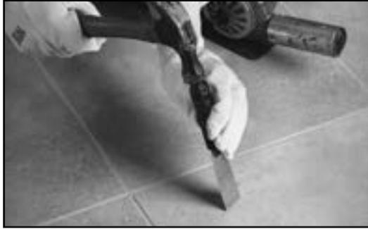
Fig. 26 - Drive a putty knife into the heated area and pry upward.
